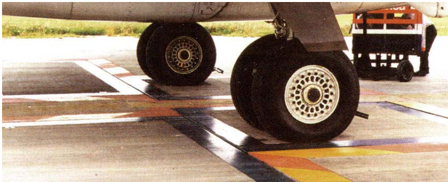
Flush in the ground installation allows for easy pull on operation at the ICAO development site in South America
